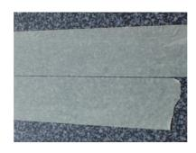
• Place the needle of the nozzle into the seam. As soon as the liquid starts to flow out pull the nozzle along the seam with a slow smooth movement, ensuring an "overspill" of about 1mm onto the masking tape.
